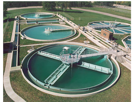
Chlorination is still used in many water treatment plants
