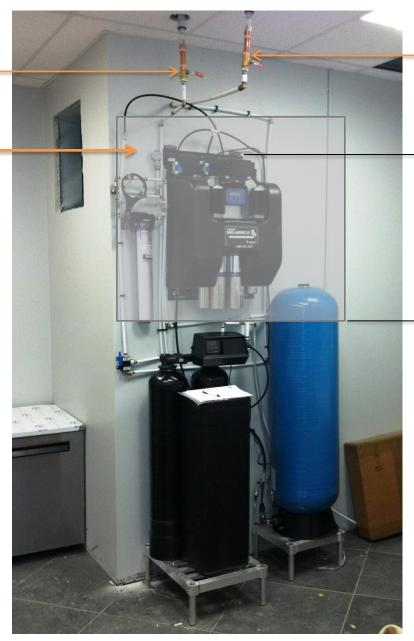
3/4" NPT shut-off valve (male or female) on the feed line required
